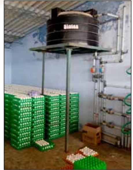
Figure 12. Having the water tank inside the house keeps the water cooler.
